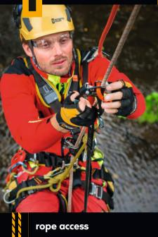
Rope access is called "royal discipline" in working at height activities. This working method is fast, effective, has little effect on the workplace and it is very quick to install nad dismantle. It is used for a wide variety of work: cleaning, painting, inspection and other working situations.
